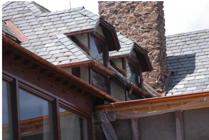
Boettcher Mansion – New ½" Slate & Copper Gutters
