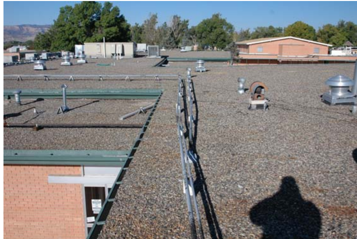
Existing Roof at Meyer Health Building – Grand Junction Regional Center
