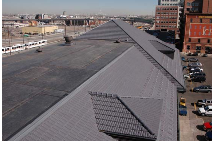
New Clay Tile Roofing – Denver Union Station
