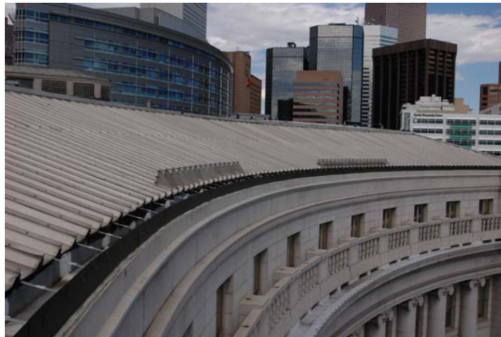
Denver City & County Building – Existing Aluminum Roof
